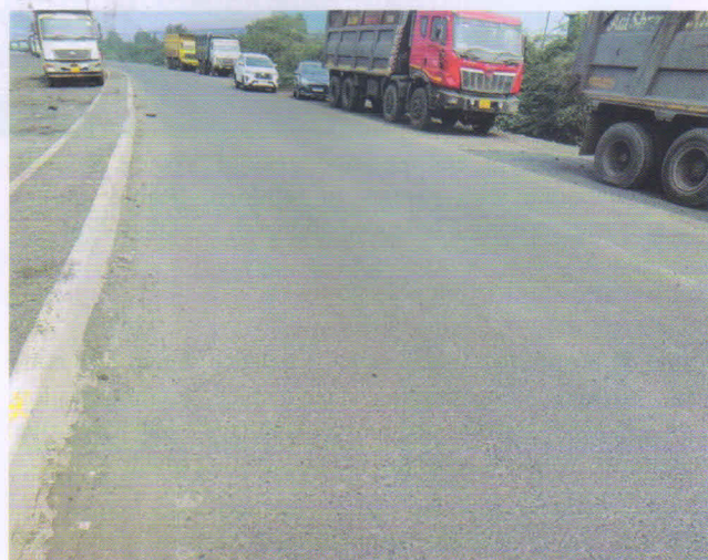
Six-lane bituminous steel slag road at Surat (Gujarat)
