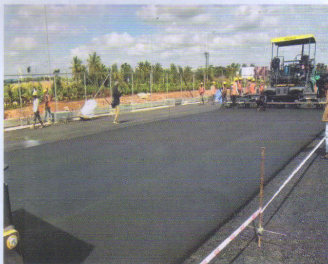
BRO constructed steel slag road at Arunachal Pradesh over a one-kilometre stretch
