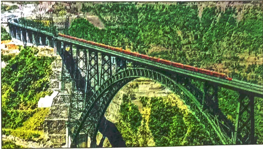
The Vande Bharat Express crosses the Chenab bridge on Thursday. (PTI)
