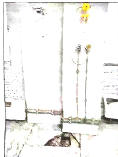
A damaged area in the ward
