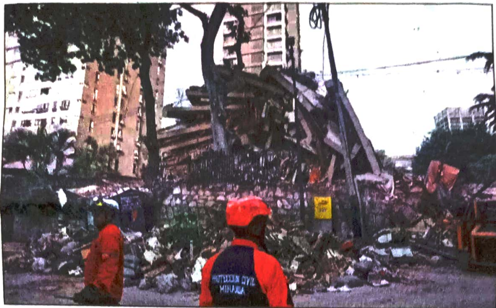
A collapsed building in Caracas, Venezuela, after the twin earthquakes on Thursday. (Reuters)
