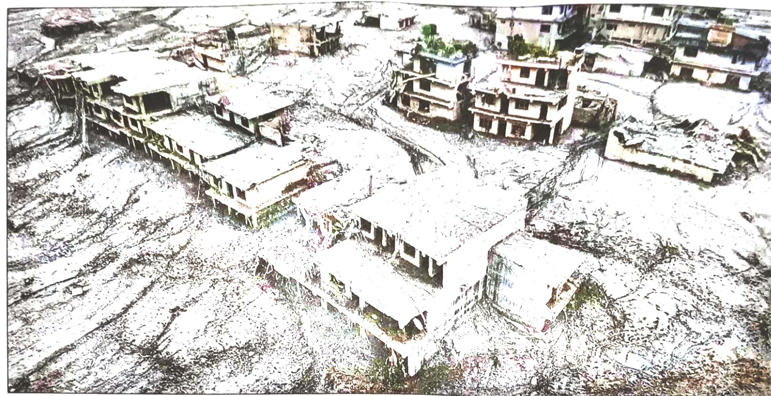
Houses covered in thick mud and debris at flood-ravaged Devighat in Nepal's Nuwakot district on Saturday. (Reuters)
