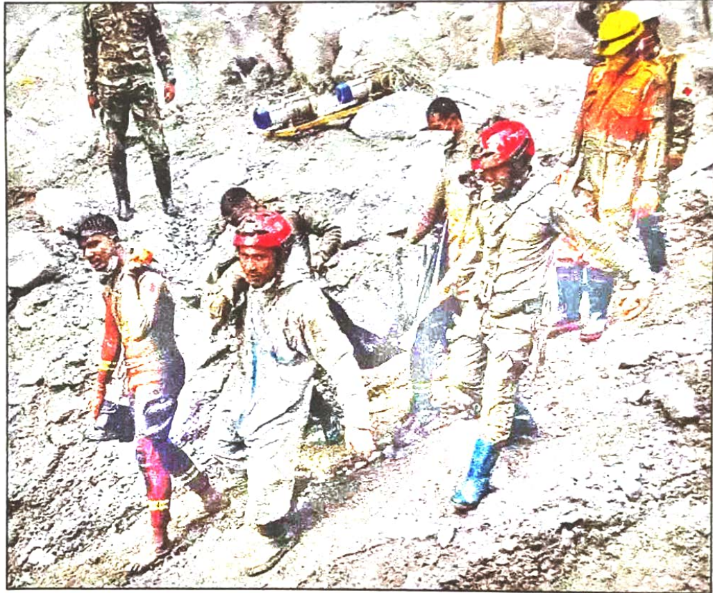
Army personnel recover a body from a tunnel of the Chilime Hydropower Project in Rasuwa, Nepal, on Wednesday. (PTI)
